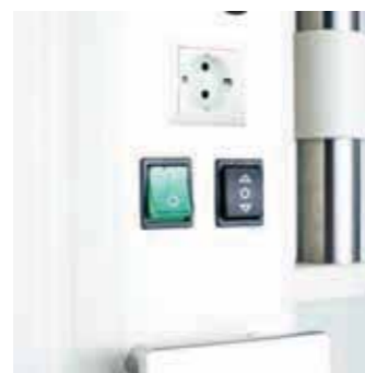
Lifting control mode 2: the control button on the distribution panel
